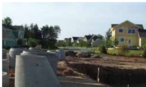
Photo: Sewer Pipes
